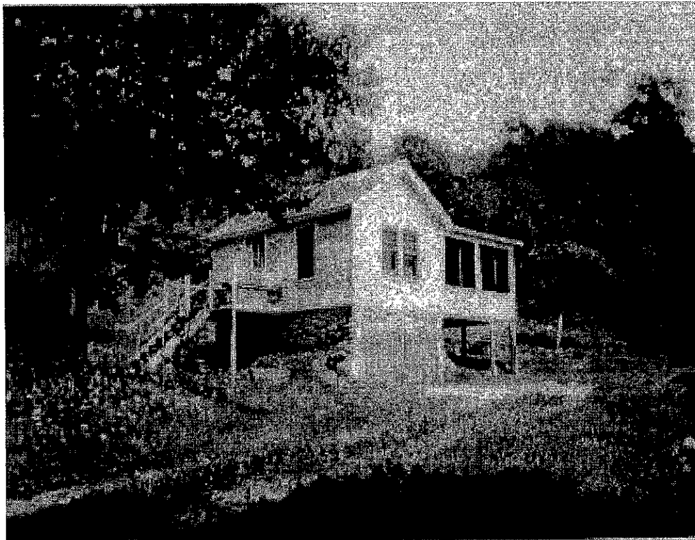
Figure 3. Franklin Williams house, Lantern Hill Reservation, 1937.
